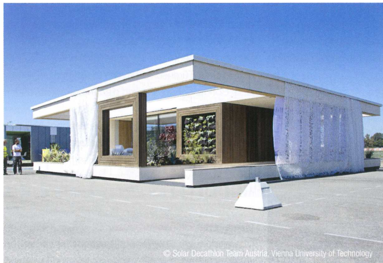
LISI, Außenansicht © Solar Decathlon Team Austria, Vienna University of Technology
